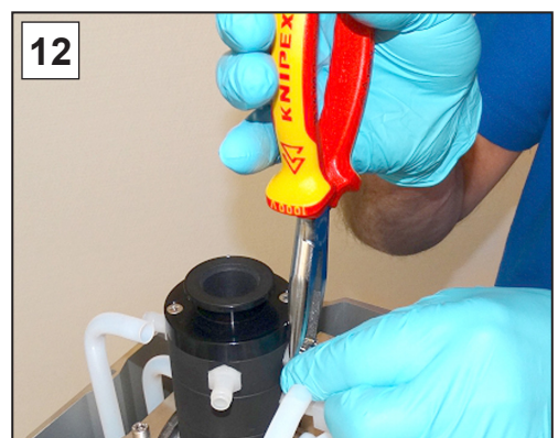
12. Secure the hose clips on the hose nozzles, e. g., with flat nose pliers.
